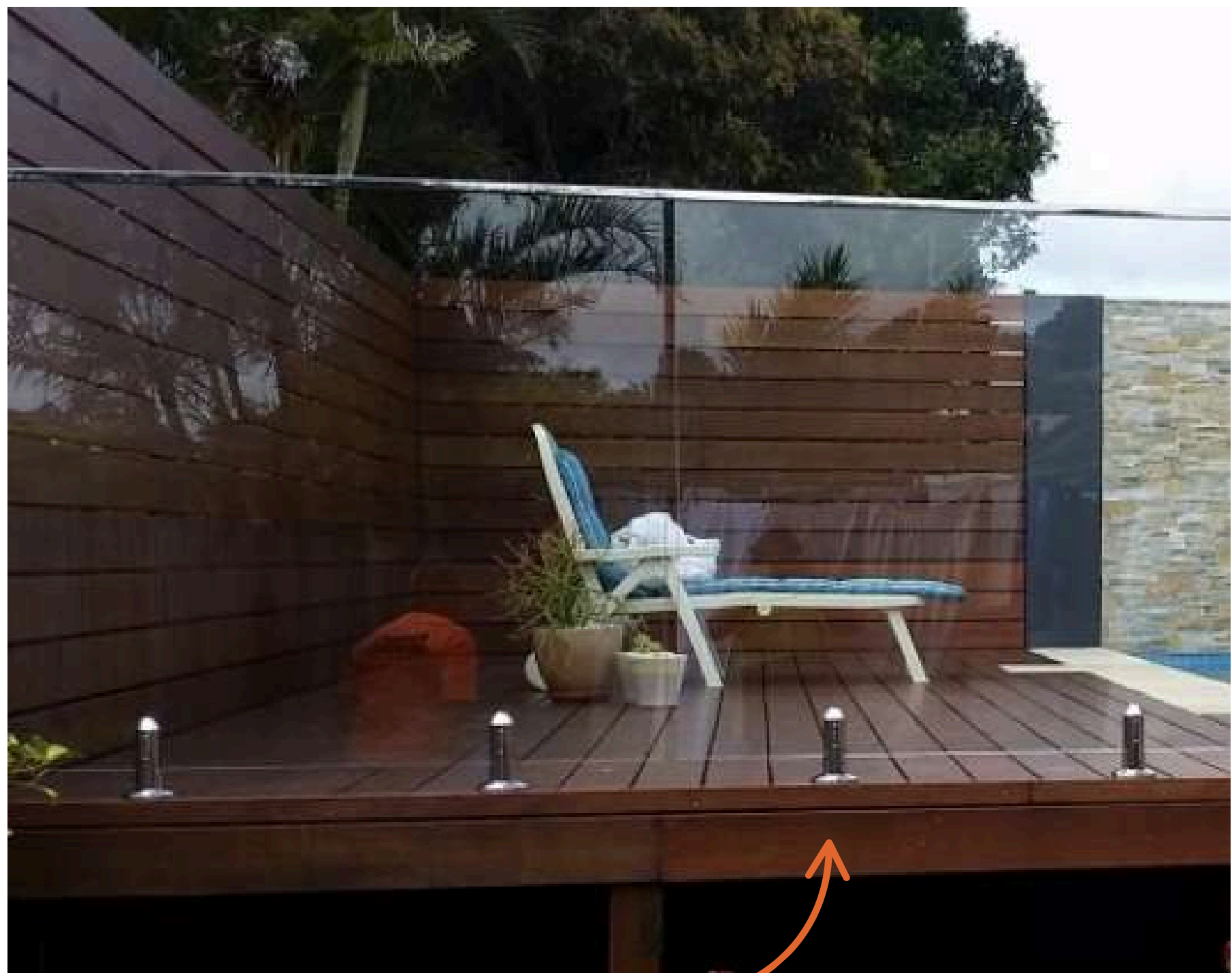
Semi-frameless glass balustrade with top mounted nano-profile handrail and spigot fixing to floor
