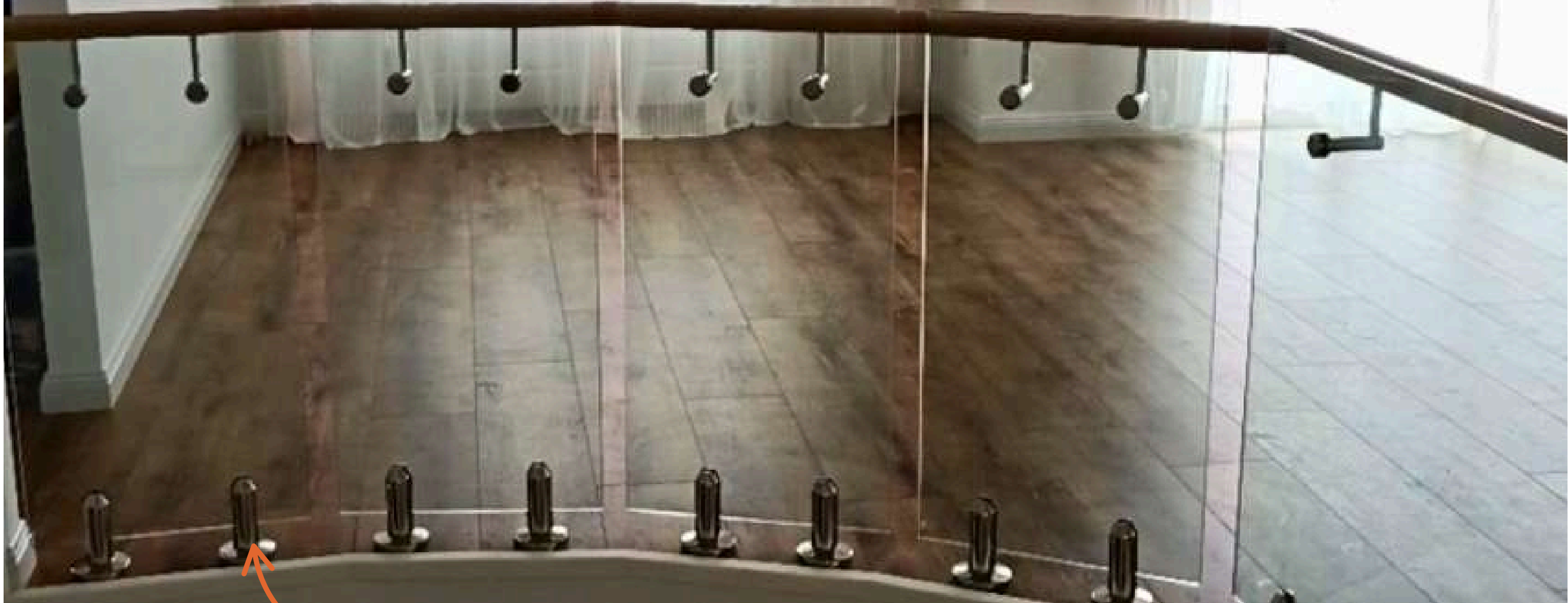
Semi-frameless glass balustrade with elbow spigots attaching handrail, and spigot fixing to floor
