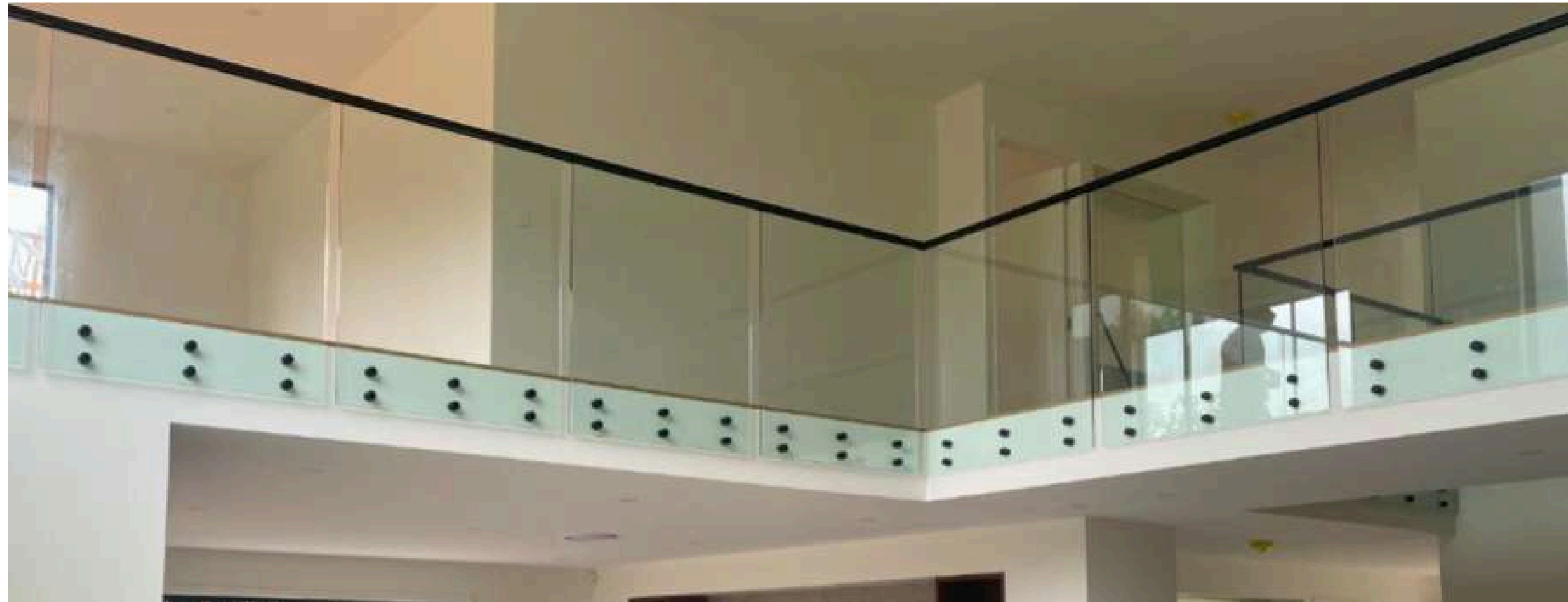
Frameless glass balustrade with elbow spigots attaching handrail and standoff mounting pins
